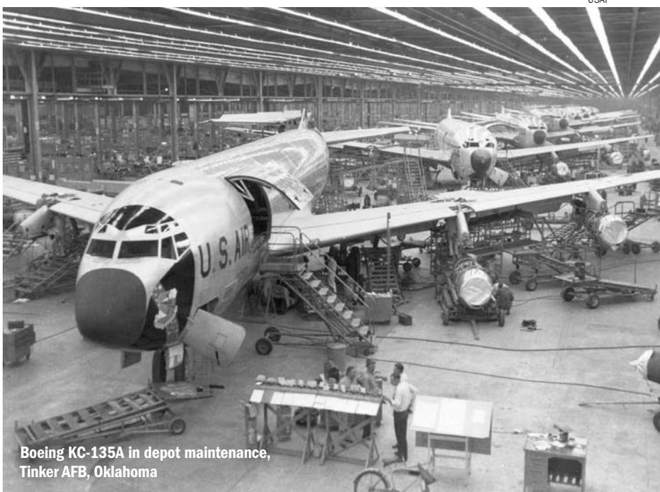
Boeing KC-135A in depot maintenance, Tinker AFB, Oklahoma
