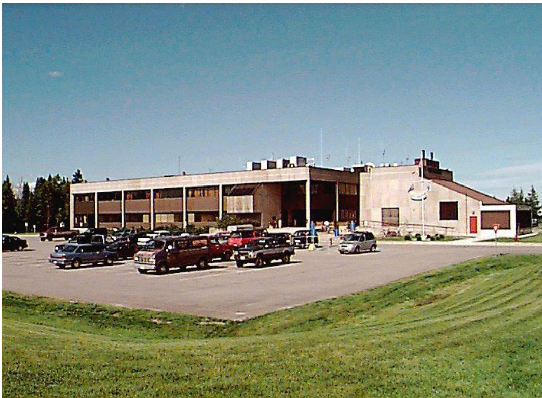
Gander Oceanic Area Control Centre Operations Building
